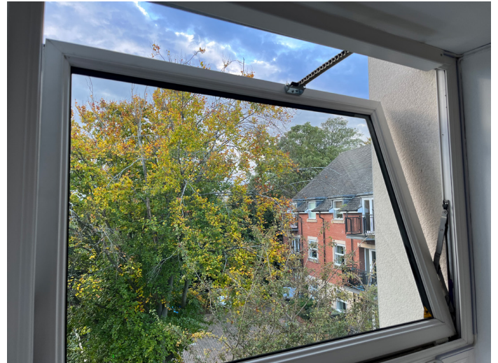
Figure 4: AOV in the open position
