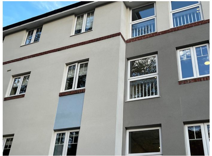
Figure 2: elevation of a residential building with AOVs – the AOVs are indistinguishable from standard windows
